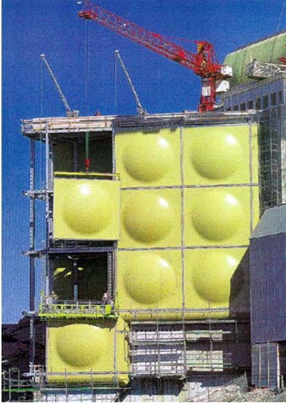
Fig. 14: Montage of a sandwich element on the steel construction
