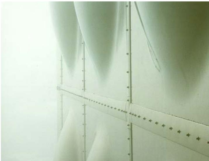
Fig. 15: Detail of the structural connection of sandwich elements on the steel construction. This Figure shows the crossing of bolted GFRP cover profiles, which are used to provide watertightness for the antenna coverage system.
