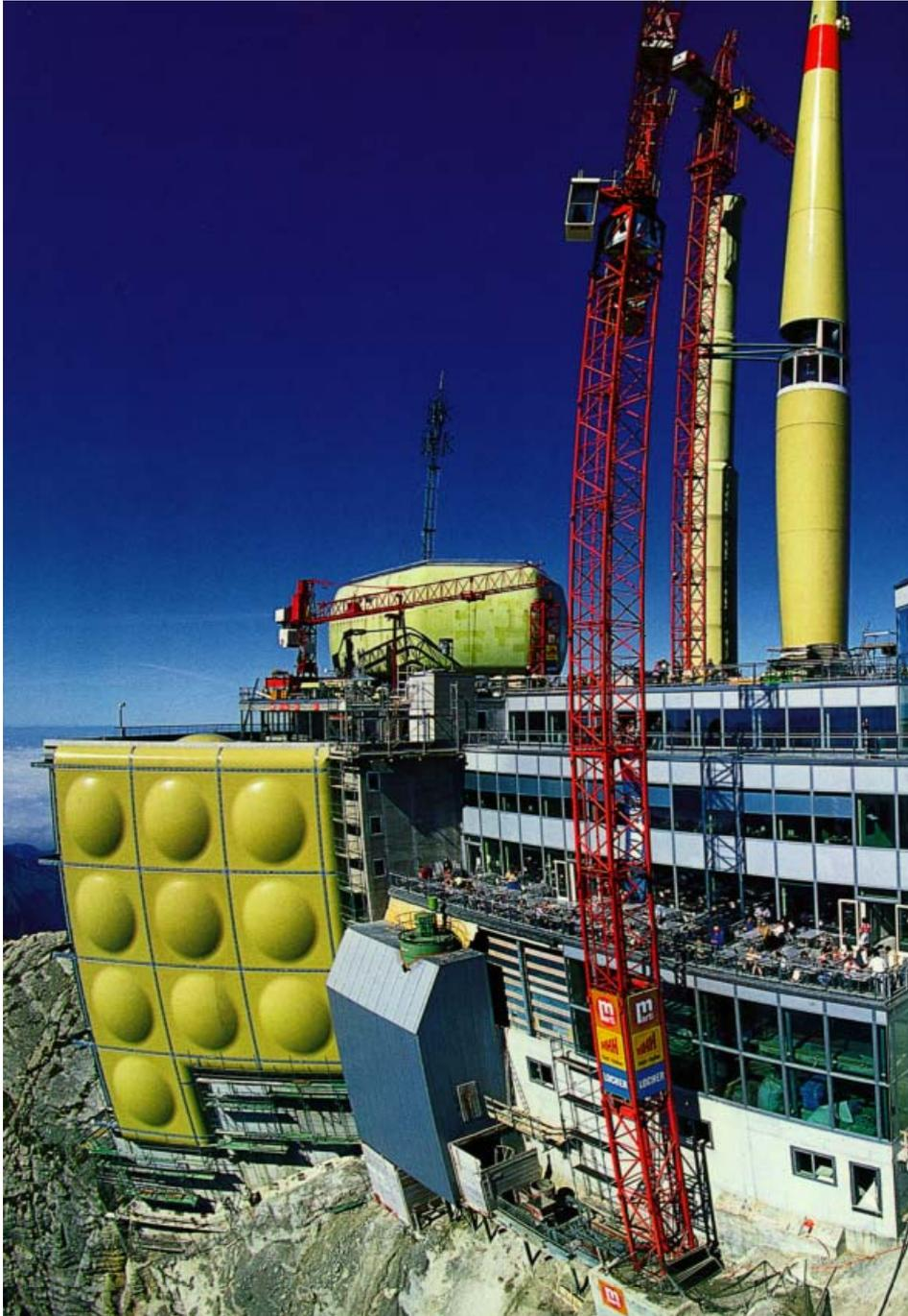
Fig. 17: Southwest view of the new antenna installations on mount Säntis. This Figure shows the new 6 m x 6.6 meter new sandwich elements and the other sandwich border elements, which together constitute the antenna coverage at the southwest side.
