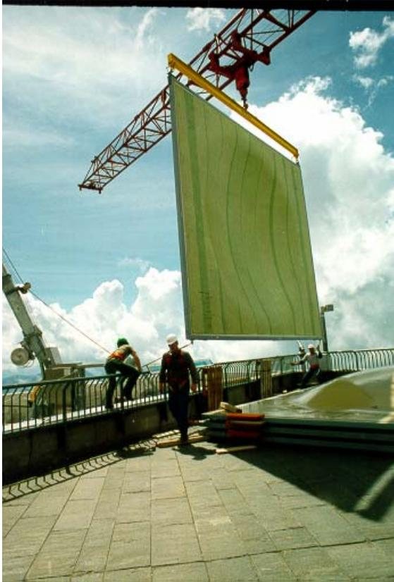
Fig. 13: Local transport of a sandwich element from the building roof to the steel framework at the side of the building
